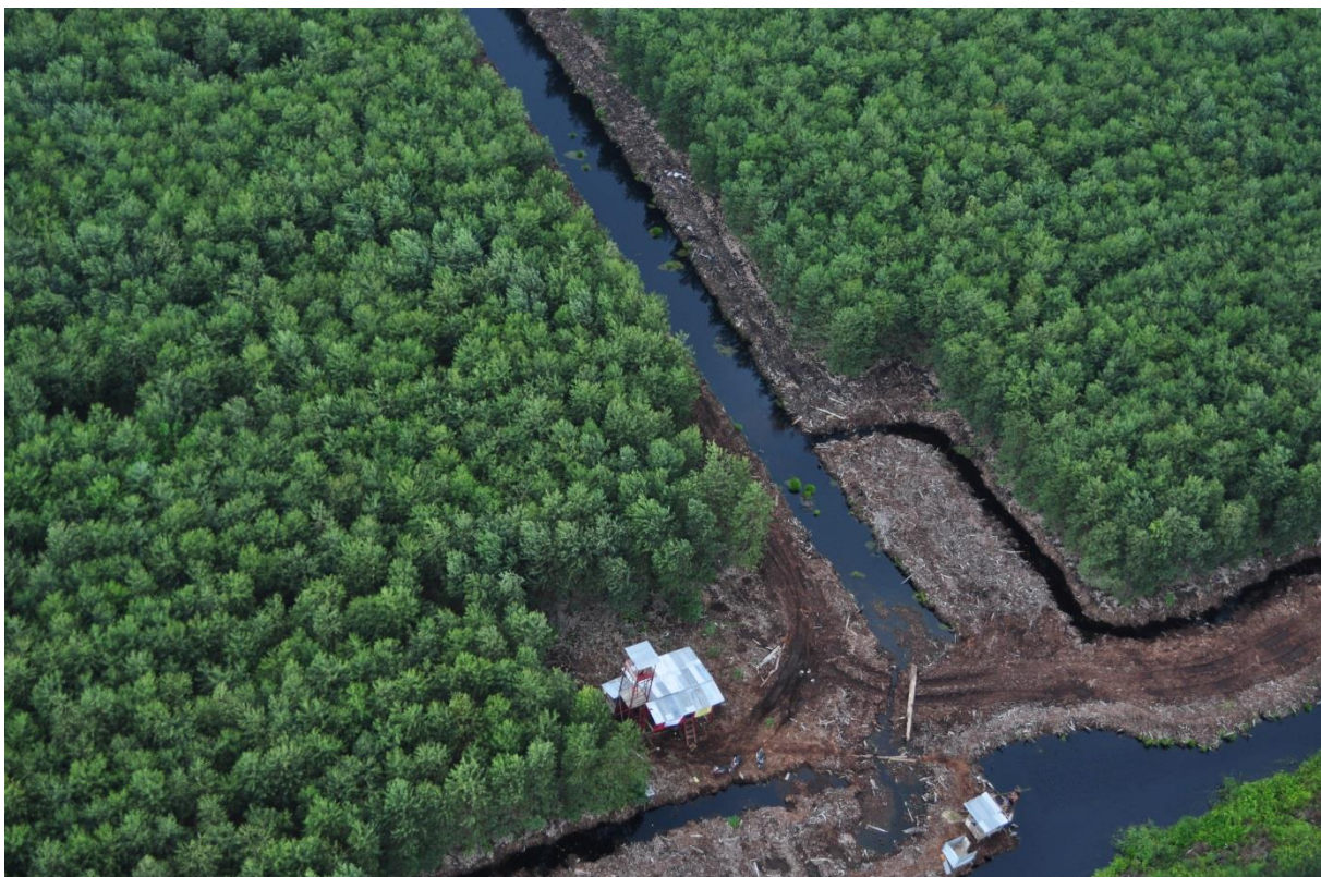
Water level regulation infrastructure in APP pulp plantation (Sumatra). Photo: Hans Joosten.
