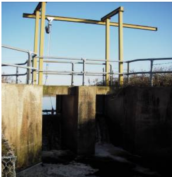
Fig. 3: Water control structures Left: concrete sluice at the point where the main ditch discharges into the river. Right: plastic overflow pipes controlling the water level behind a clay dam. (photos O. Bragg).
