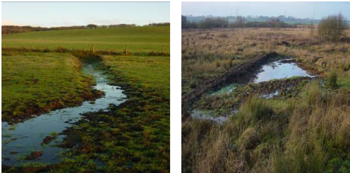
Fig. 4: Water management work at the eastern side of Cors Erddreioniog after 1998. Left: stream emerging from a buried agricultural field drain which has been severed at the site margin in order to allow base-rich water to flow into the peatland. Right: a new peat bund holding back water in a small pool on one of the north-south ditch lines. (photos O. Bragg).
