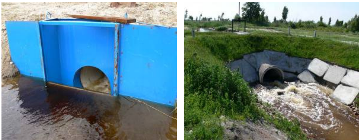
Fig. 18: Sluice constructions at Zvanets mire
