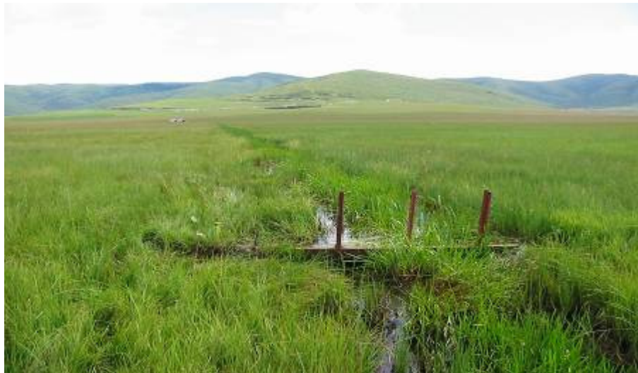
Fig. 45: Wooden plank dam
