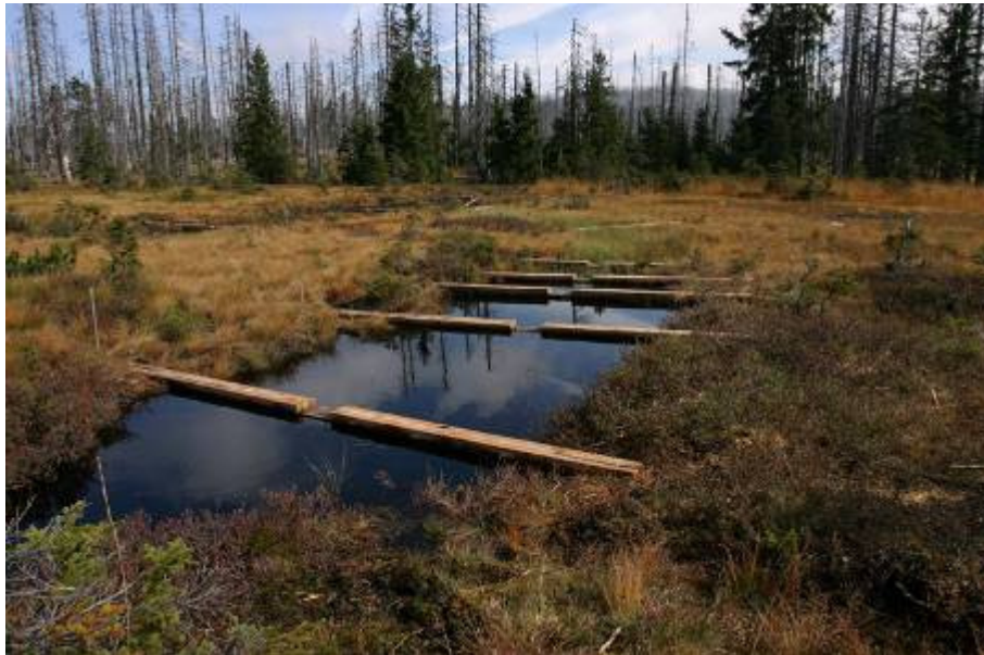
Fig. 14: Cascade of dams along a ditch
