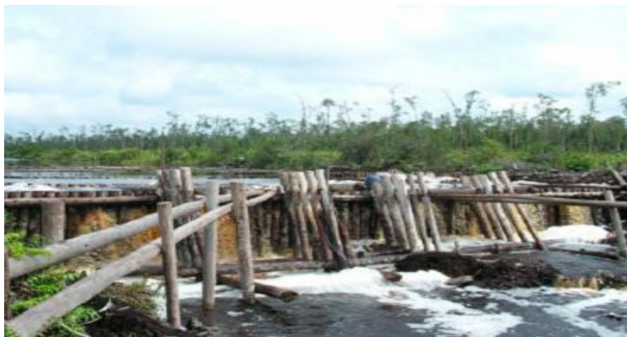
Fig. 29: Large wooden dam, filled with stones
