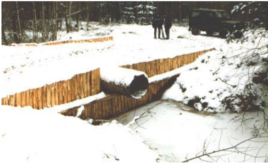
Fig. 23: A single dam, designed to double as a bridge (photo Ecological Centre Dront)
