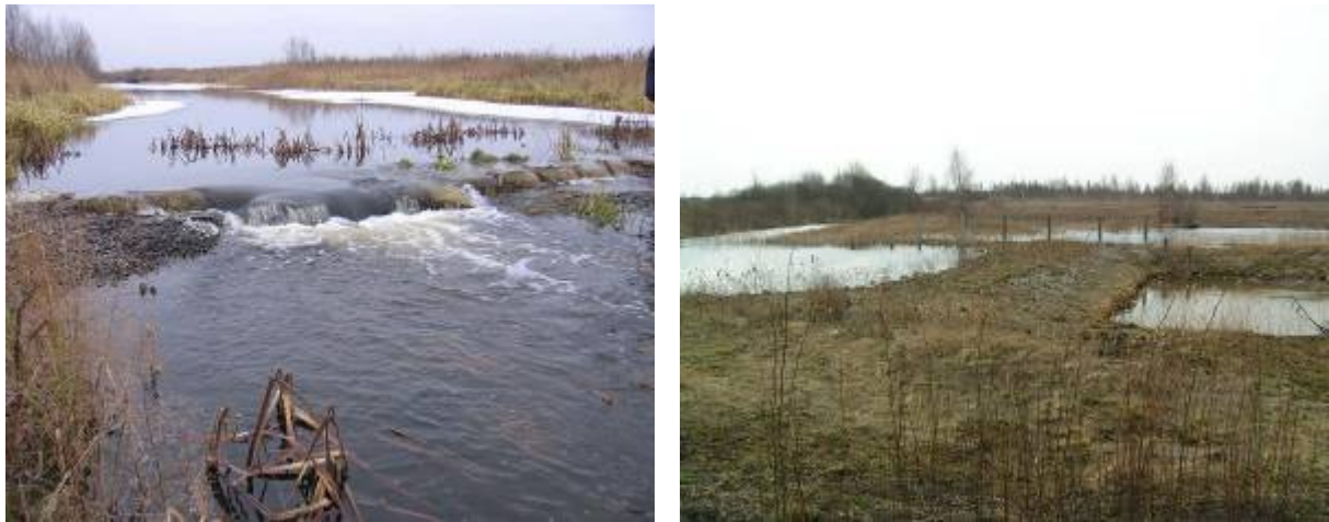
Fig. 17: Dam constructions at Zvanets mire
