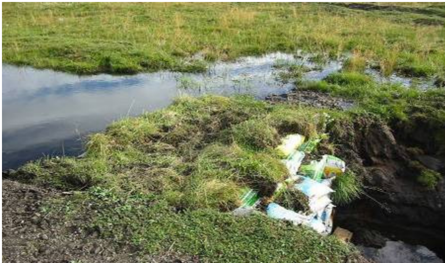
Fig. 38: Dam made of plastic bags, filled with peat
