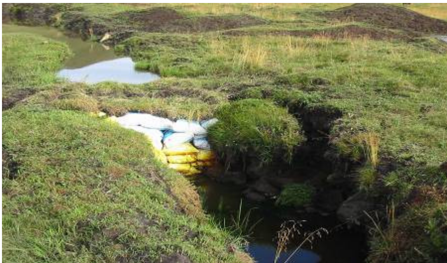
Fig. 39: Dam is backing up water
