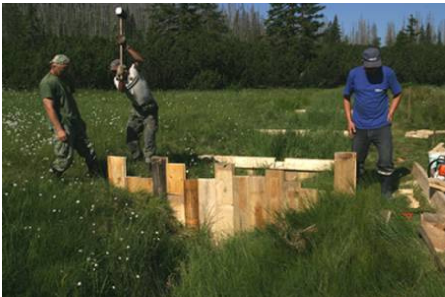
Fig. 13: Installation of wooden plank dams with overflow
