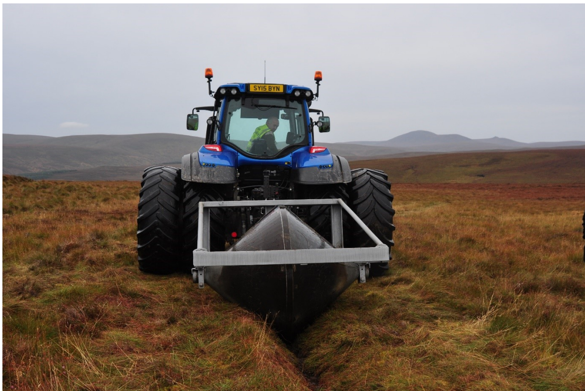
Ditch reprofiling in the Flow Country. Photo: Hans Joosten.
