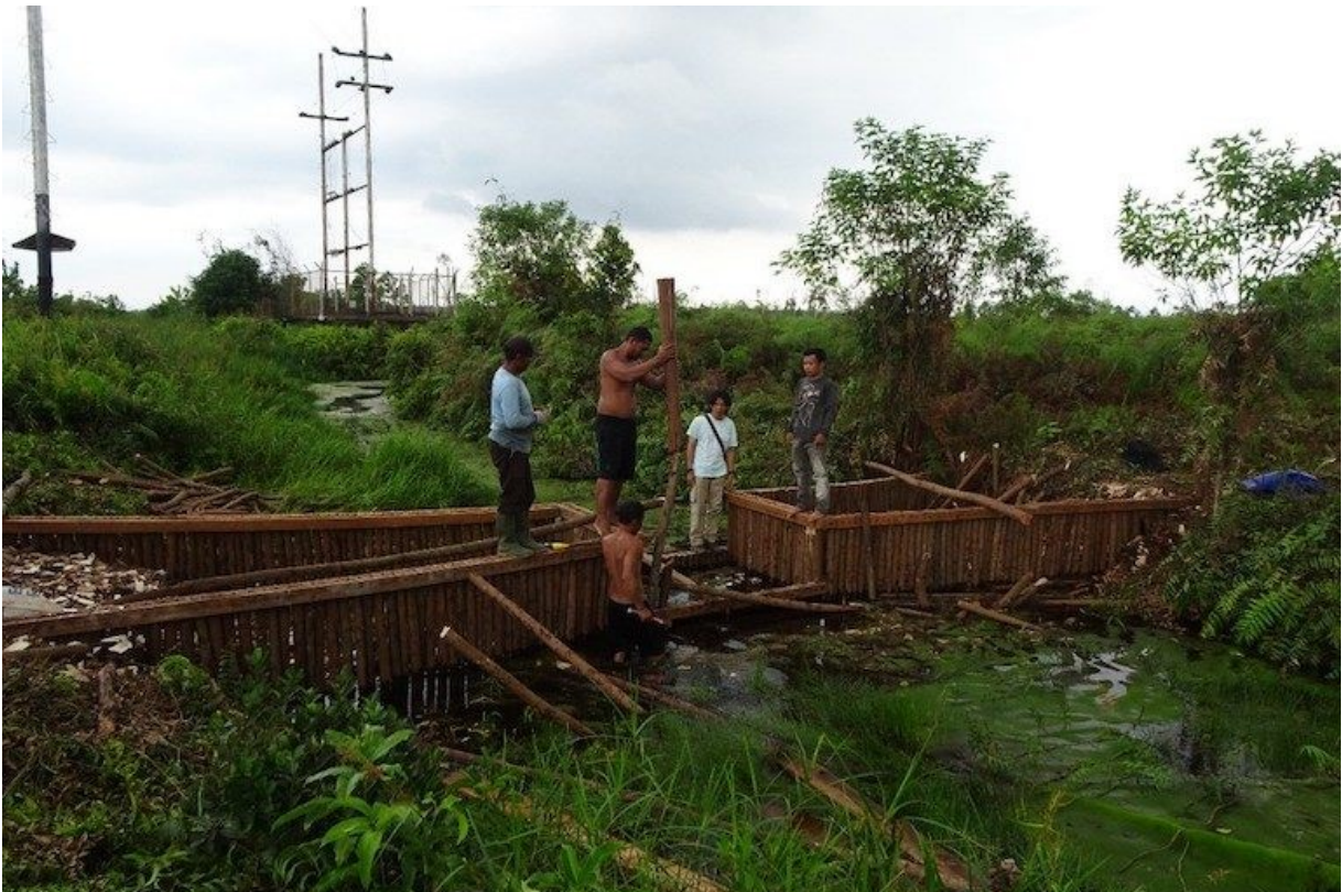
A group works to block a canal made to drain a peatland near Dayun village in the Sumatran province of Riau, Indonesia. Photo: Wetlands International.
