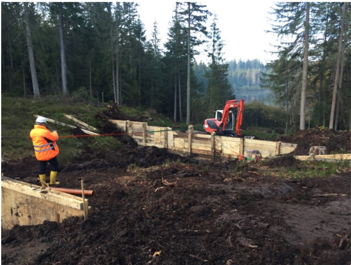
Ditch blocking in 2018 to restore the natural dynamics of the bog. Photo: SP-Canton du Jura
