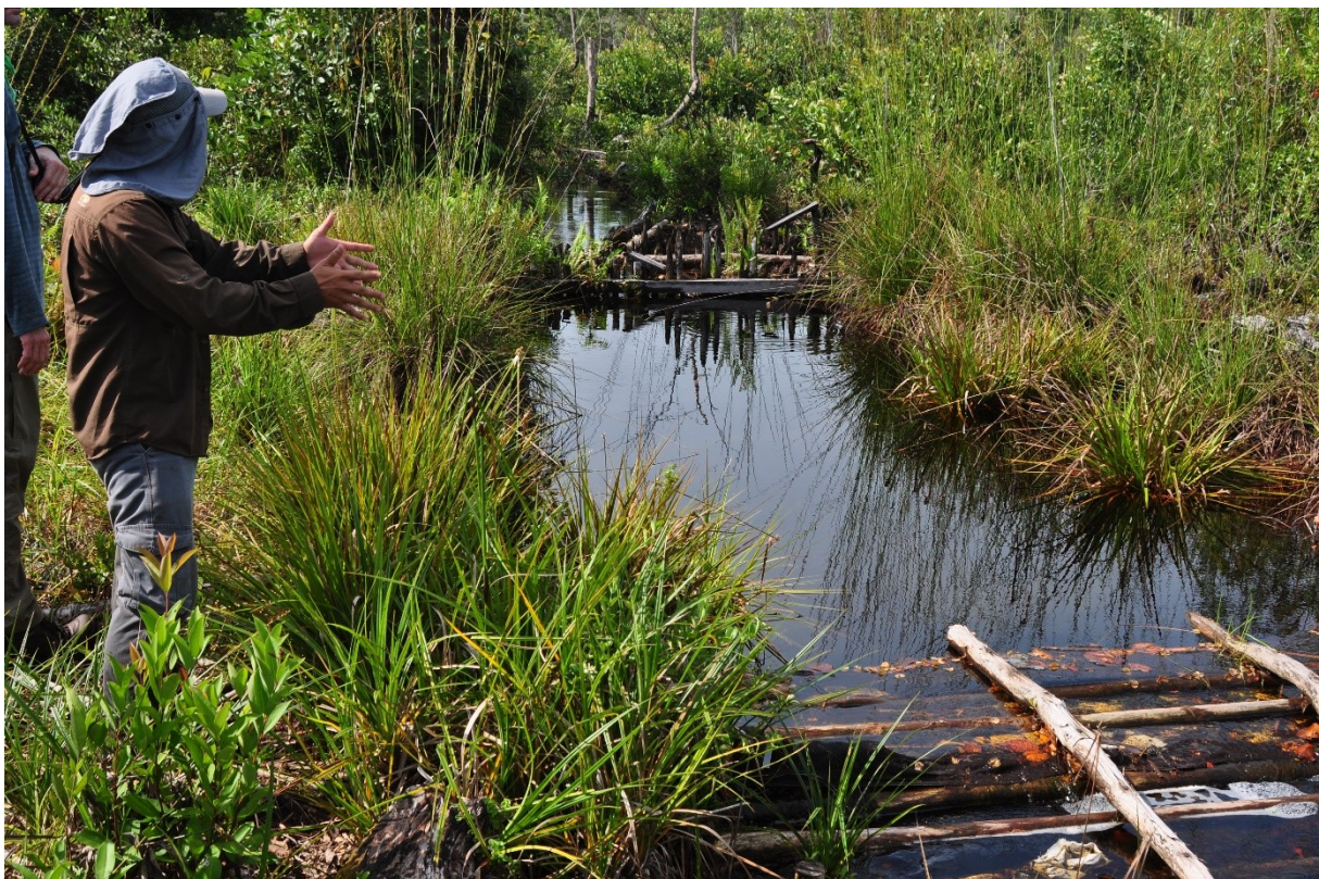
Simple ditch blocks in Central Kalimantan peatland. Photo: Hans Joosten.
