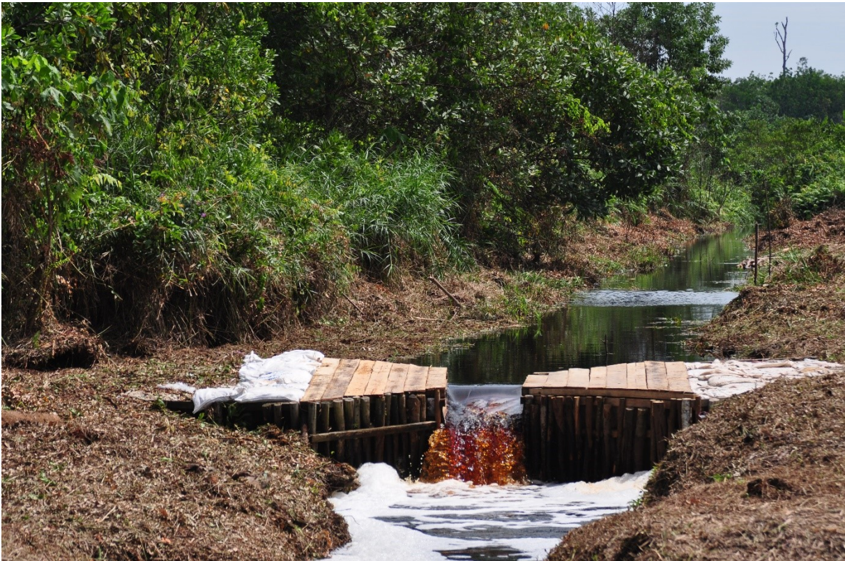
Peatland rewetting in Riau, Sumatra, Indonesia. Photo: Hans Joosten.
