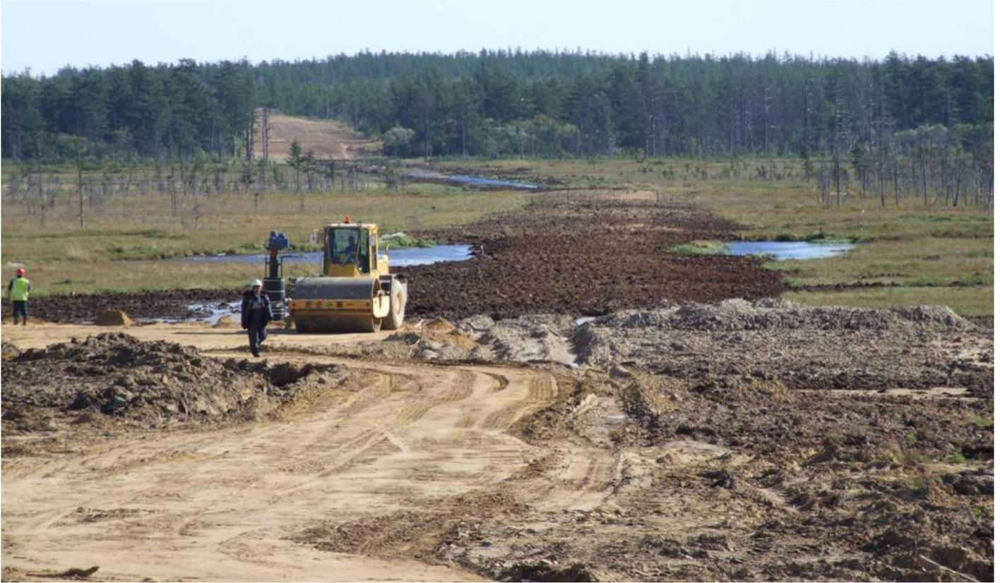
*Cutting the natural flow of water in mires by pipeline construction in Sakhalin (photo Andrey Sirin).*
