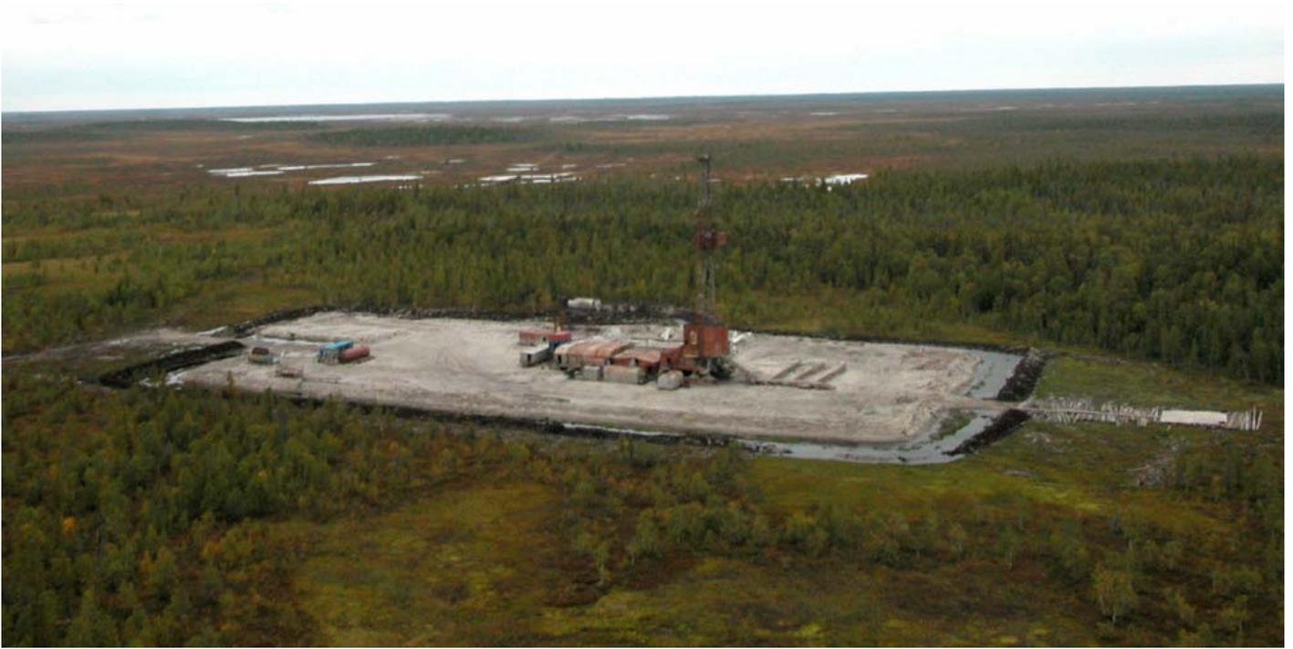
*In highly paludified areas oil and gas drilling towers are often put directly in the mire after building a platform and protective dams (West Siberia; photo: Andrey Sirin).*
