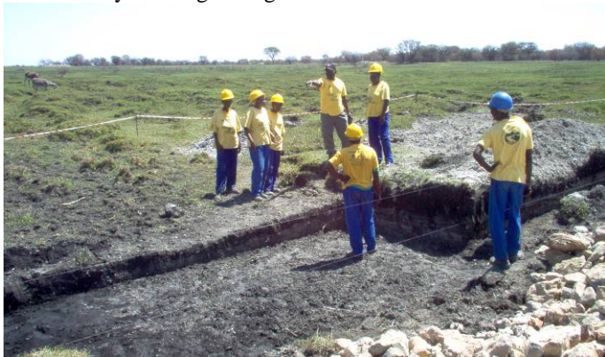
Thilivhali Nyambeni, an IMCG member instructing a Working for Wetland team on how to build a small weir in the Molopo mire to arrest erosion and to lift up the water table. Thilivhali started off as a student project manager. He is now, 8 years later the Provincial Coordinator of Working for Wetlands in the Free State Province of South Africa.
