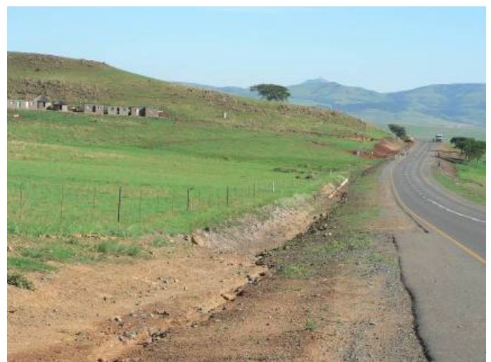
Figure 4: Secondary impacts on other wetlands such as from roads to the construction sites. This road is effectively draining the upstream part of a seasonal wetland.
