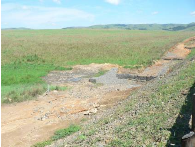
Figure 5: Failed attempts to rehabilitate. Note the sheet erosion still occurring in the foreground and rubble behind the gabion structure. This structure has recently collapsed, resulting in more erosion of this wetland.
