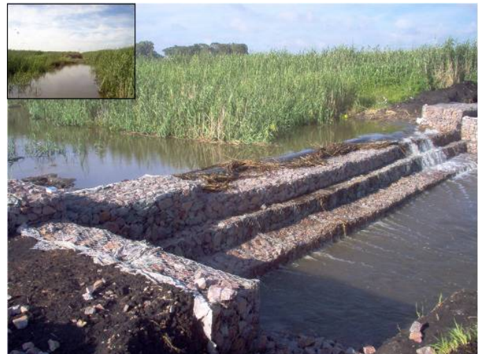
Drain blocking with a gabion weir, effectively lifting up the water table and de-activating the erosion potential (insert).
