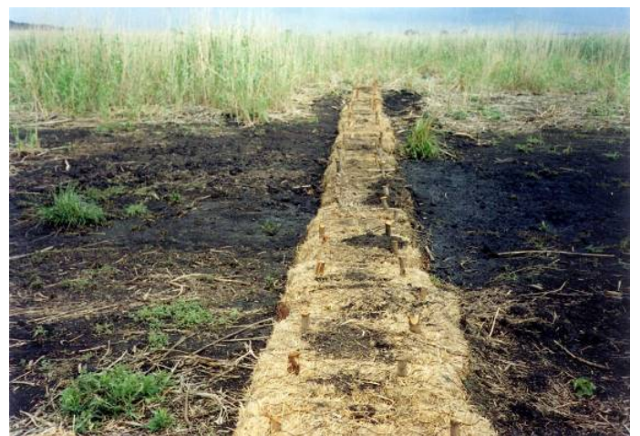
Hay bales are used to slow down flow in a shallow erosion gully in the peat. The bales were later replaced with gabion structures or earth dikes.
