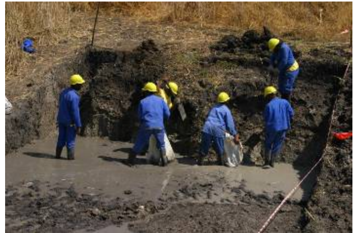
Contractors busy with the excavations for the gabion weir shown in the previous photo.
