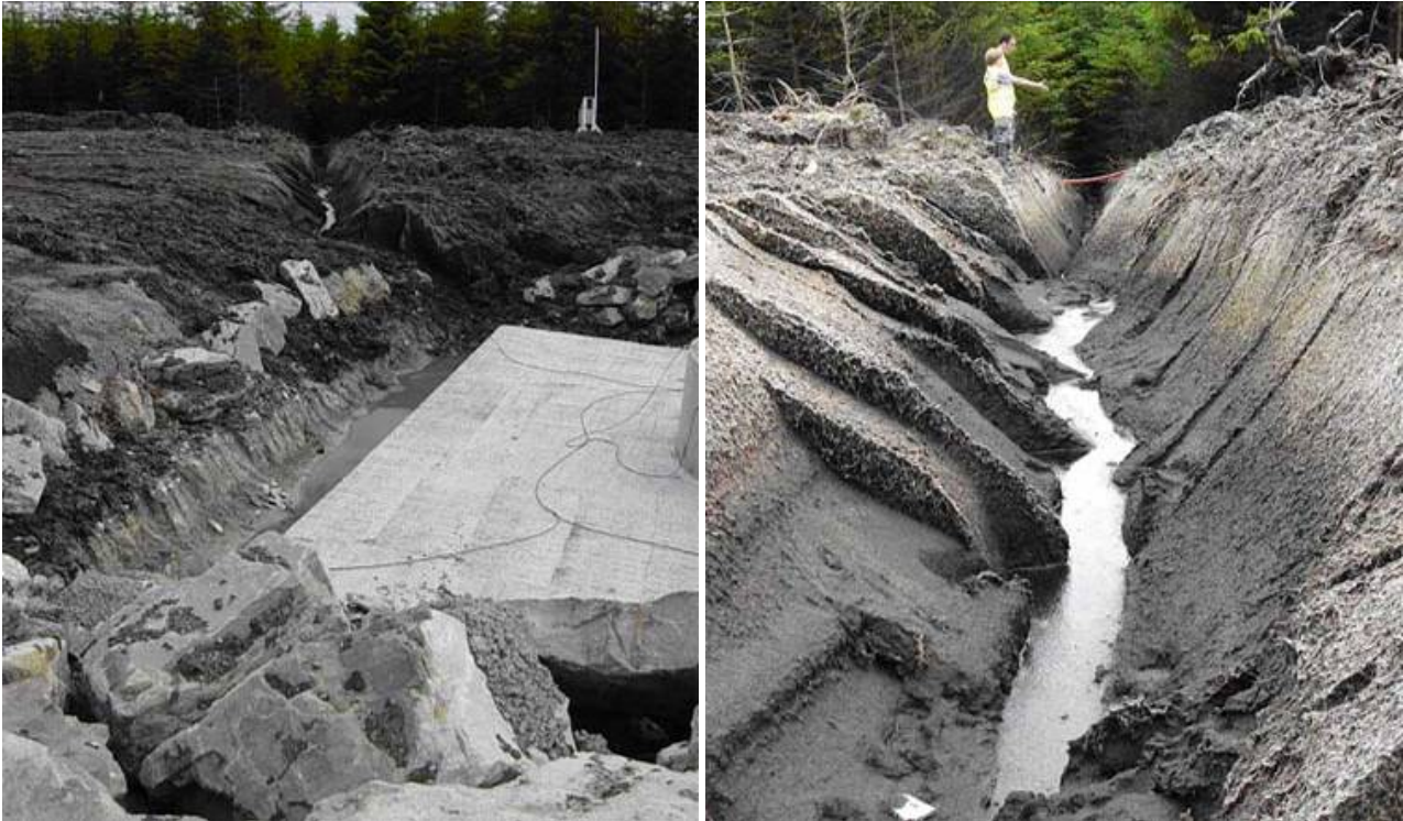
Plate 5. Drain dug to release water from the excavation for Turbine 2. Note the rock reinforcement that is required to stabilise the sides of the excavation and the telemetric monitoring equipment in the background that will detect any movement of peat which, at this location, would descend directly onto housing in the village of Derrybrien.
