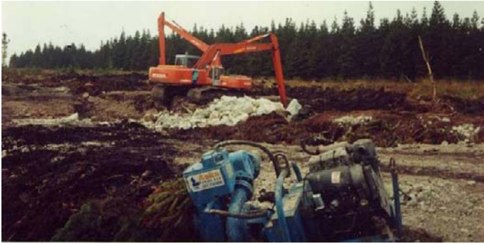
Plate 4. The site of Turbine 68 shortly after the bog slide, showing the two abandoned excavators and a disconnected water pump. The position of pump suggests that it could have been used to pump water from the excavation. (Photograph: M. Collins).
