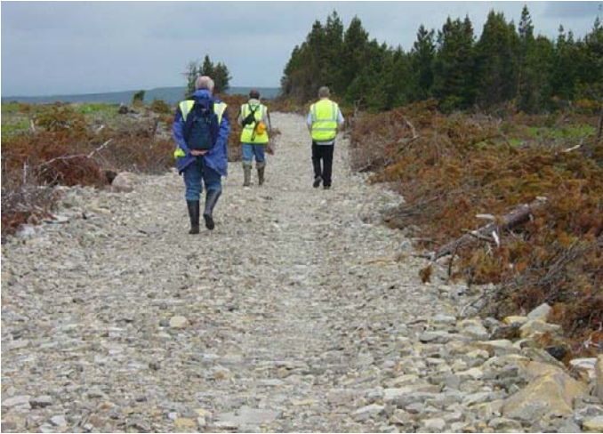
Plate 1. Floating road at Derrybrien Windfarm. The effect of loading the raft of brushwood and timber with 1.5 m of rock aggregate is already evident from the angles of the tree trunks protruding at the sides of the road; it seems questionable whether this construction will continue to 'float' throughout the 25-year projected lifetime of the windfarm.
