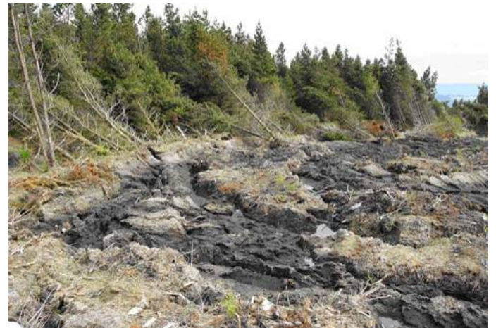
Plate 3. Looking downslope from Turbine 68 on 08 June 2004. The peat appeared to have separated from the plantation along plough furrows to form long ribbons that were progressively drawn into the slide.
