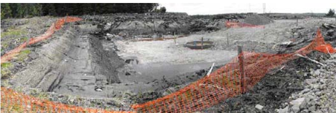
Plate 2. Two examples of turbine foundations at Derrybrien Windfarm. Above: concrete pad and steel base-can before addition of overburden at Turbine 23. This site is in shallow peat, the upper face of the concrete pad lying below the level of the peat-mineral interface. The purpose of the blue caps inside the can is to protect the electrical connections for the rotor, and the copper wire draped around the pad is the turbine's earthing net. Below: the foundation for Turbine 67, in deep peat, after backfilling with overburden. The upper rim of the can remains just visible above the finished hardcore surface. The area of peat removal is very much larger than that of the 15-metre-square concrete pad, and the permanently exposed peat faces on three sides of the excavation are already showing signs of drying-out and cracking.
