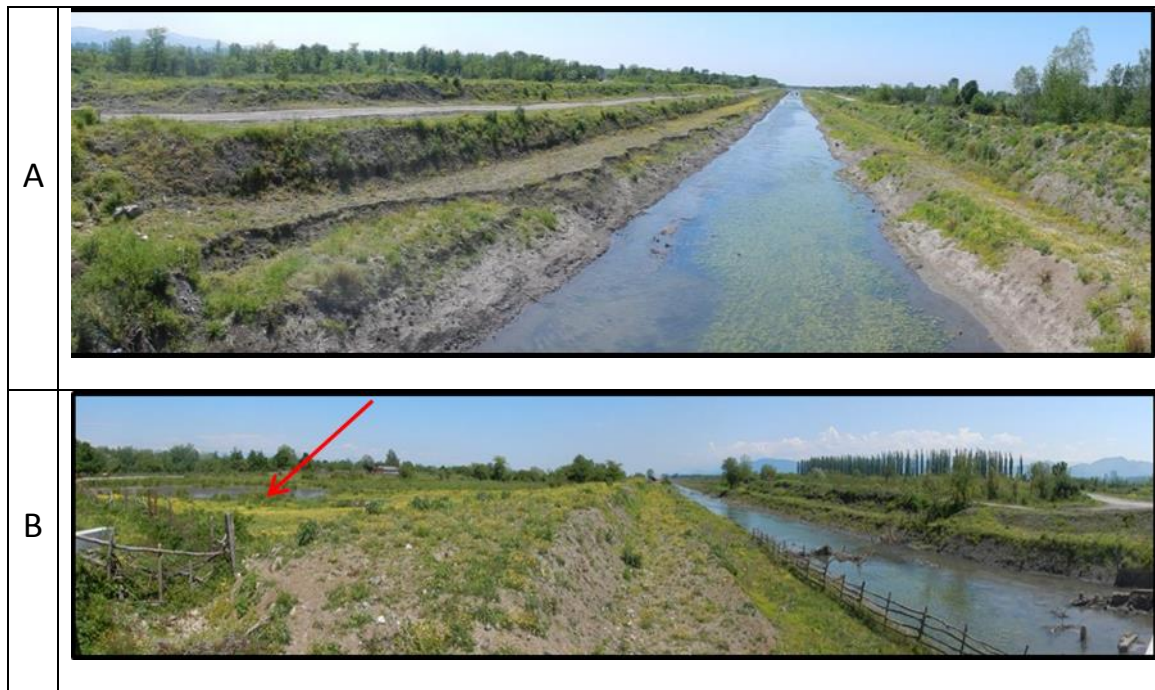
Fig. 4. Photo A shows a 4-6 meter deep drainage channel, aimed at rapid discharge of surface water in order to avoid long term flooding in agricultural areas. On the left it can be seen that the pressure of groundwater is causing the channel wall to slip into the channel. However, these costly measures do not seem to have any effect, since a permanent wetland is found within 50 meters of the channel. The channel only succeeds in transporting large amounts of floodwater to the coast, but it hardly influences water levels in the direct agricultural surroundings.
